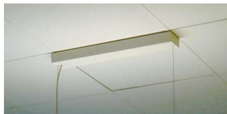
CEILING CUP CC 60 CM BETWEEN THE WIRES
